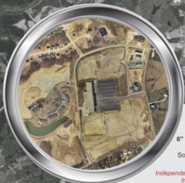
1999 Color Photos 6" & 12" resolution Source: GRW Aerial Surveys, Inc. Independence Town Center Independence, KY
